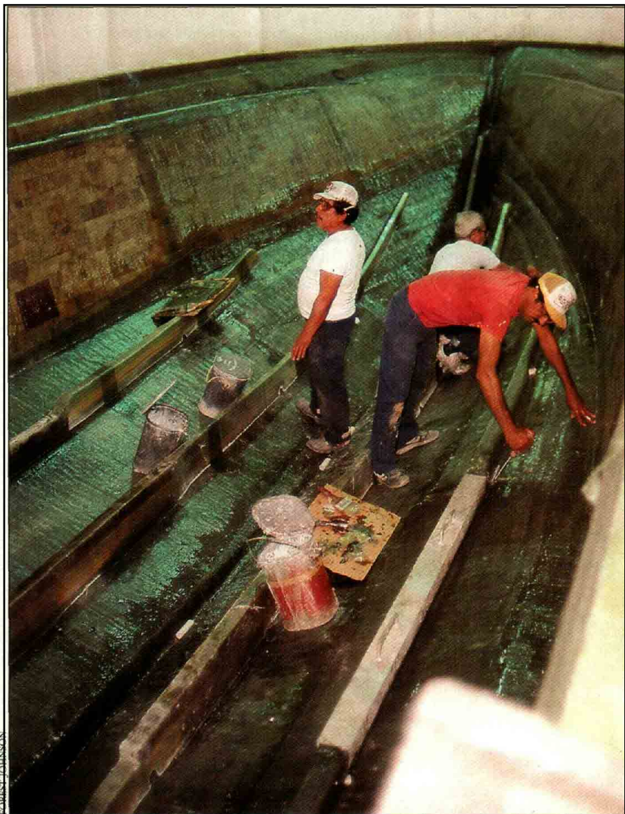
Many builders have their best laminator make up test panels under ideal conditions, forgetting that what happens on the production floor, where the boat is actually built, is something altogether different.
